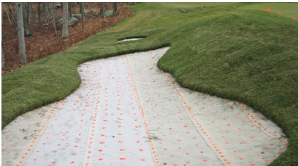
A golf course bunker being sodded with Black Beauty.
